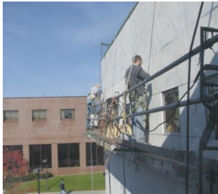
Exterior marble repair by Brick-Well Masonry of Youngstown.
