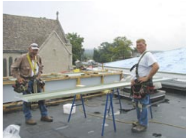
Butler roof repair by Related Metals, Inc. of Youngstown.
