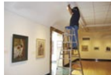
Museum preparator Wayne Gruver is seen installing new LED fixtures in the Butler's Giffuni Pastel Gallery. To date, most of the museum's permanent collection galleries have been refitted with the new lighting which will not only save energy, but will also help to preserve the valuable works of art in the Butler's holdings.
