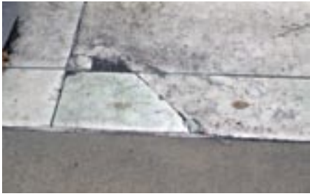
Marble sidewalks have incurred damaged from freezing and thawing over many winters.
